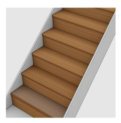
You can now repeat the process down the flight, riser first followed by tread. If there is a turn on the flight or a larger step you can use our tread extension kit at this point.
